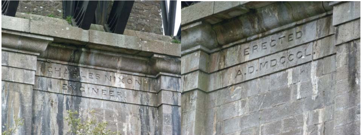
Figure 2.24: Details of Engineer and Contractor inscribed on piers
