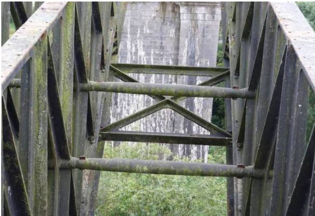
Figure 2.19: X-shaped cast iron bracing and transverse wrought iron tie rods
