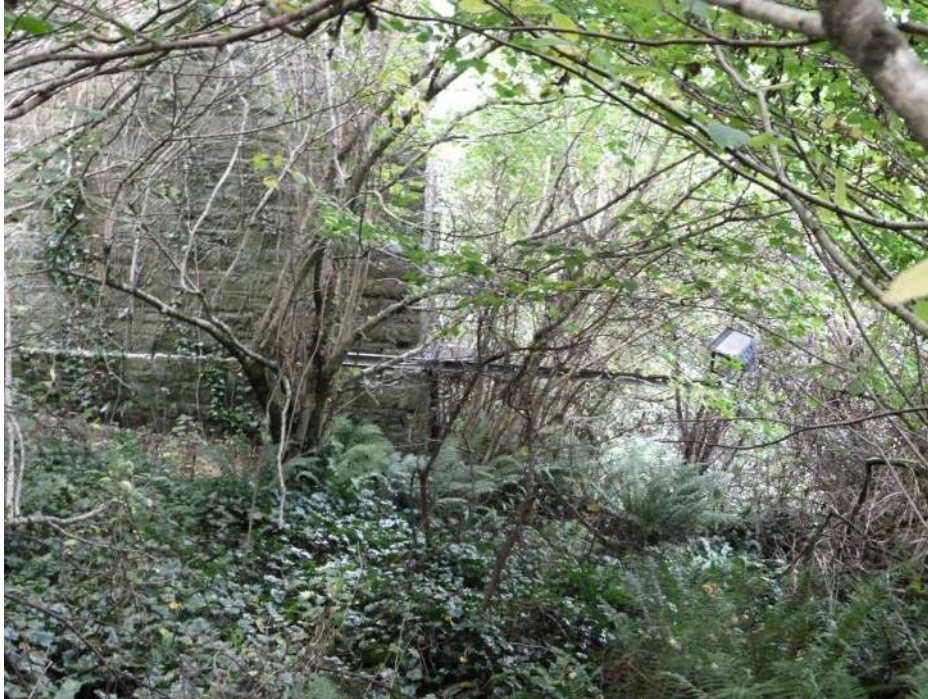
Figure 3.19: Bridge up-lighting attached to pier
