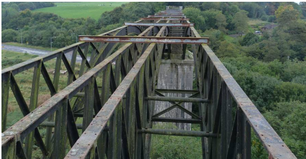
Figure 2.4: Current condition of bridge surface
