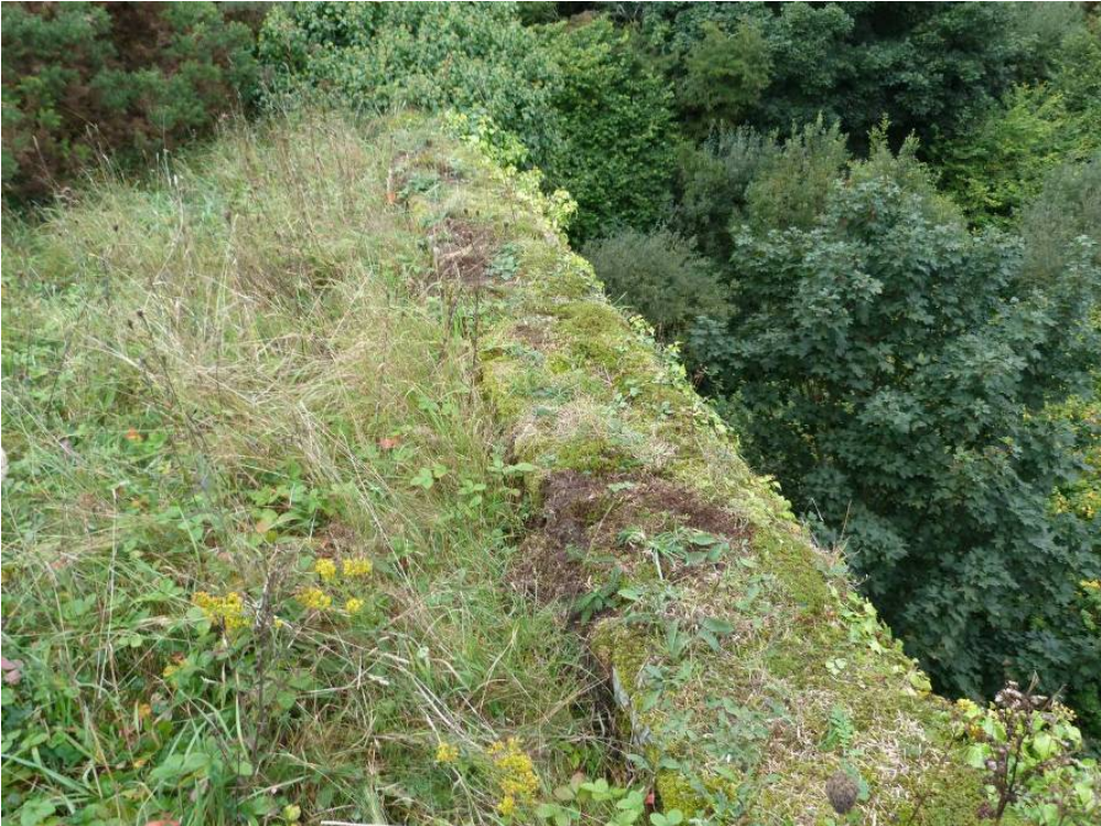
Figure 3.4: Northern masonry parapet wall
