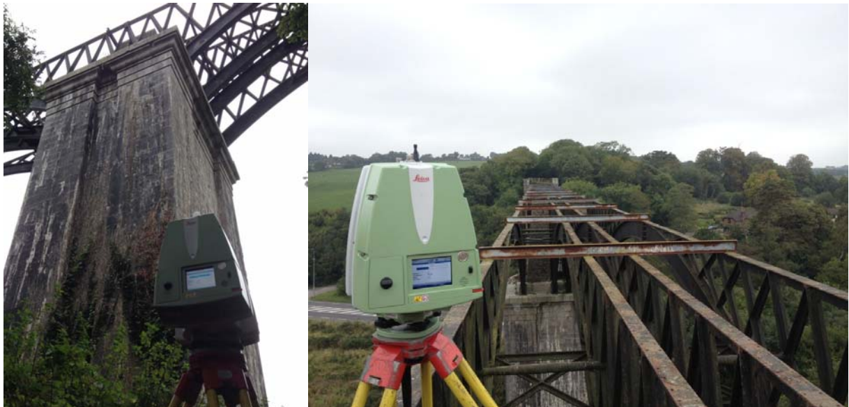
Figure 2.29: 3D laser scanning of Chetwynd Viaduct in operation
