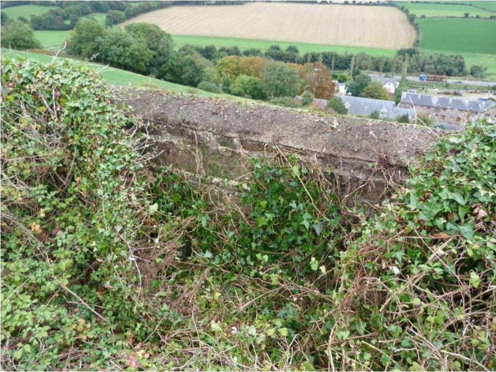
Figure 3.5: Southern masonry parapet wall
