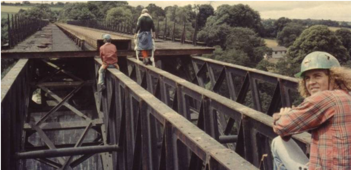
Figure 2.6: Bridge deck partly removed, circa 1970
