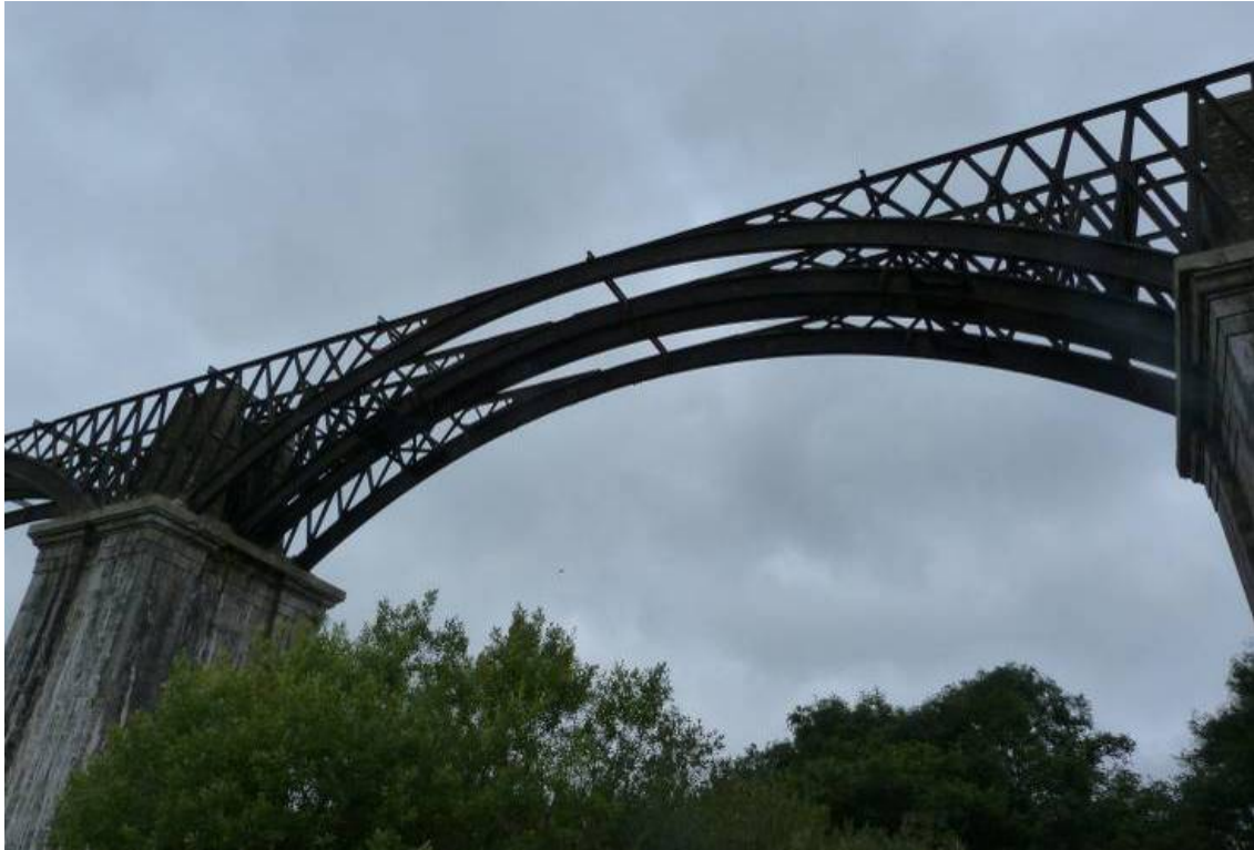
Figure 2.7: Cast iron arched ribs
